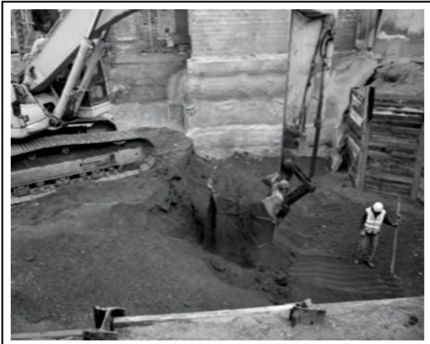
(f) Machine work at the edge of excavation
