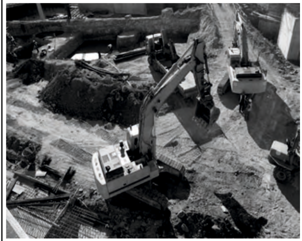
(d) A typical view of excavation work at construction site
