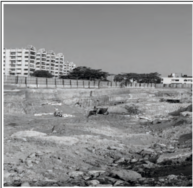
Fig. 4. (a) A typical view of excavation
