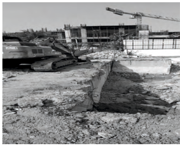
(c) Machines are at the edge of excavation
